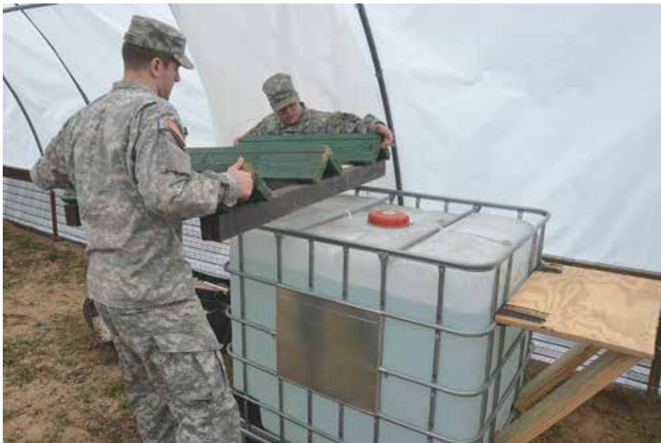
Kyle Harrell '17 (foreground) and Nate Whitmer '17 install raised beds on top of the fish tank in the aquaponics project at Natural Bridge. – VMI Photo by Stephen Hanes.
